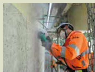
ひび割れ補修
